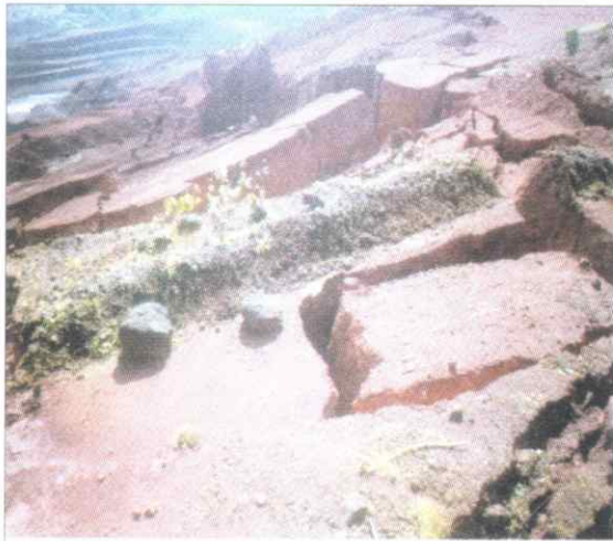
Fig 1. Pit slope failures in iron ore mines, Goa, India
