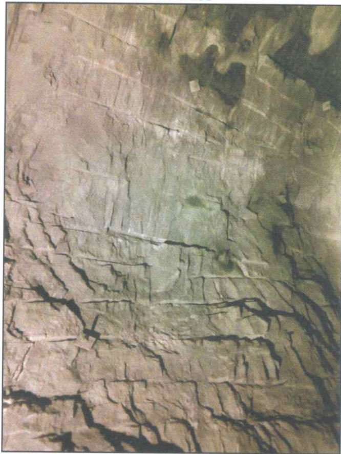
Fig. 6 Tunnel profile with maximum half-cast factor after application of new blasting techniques at LNPHEPP
