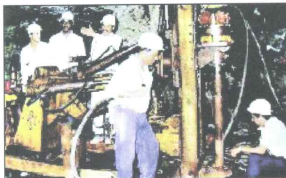
Fig-5 : Drilling at Hutti
