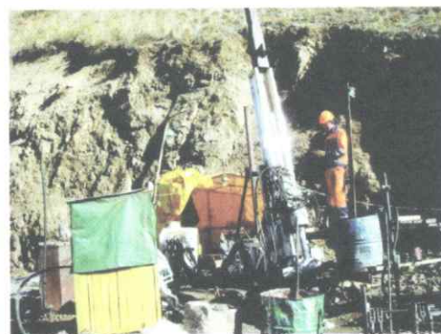
Fig-6: Drilling at Chaarat
